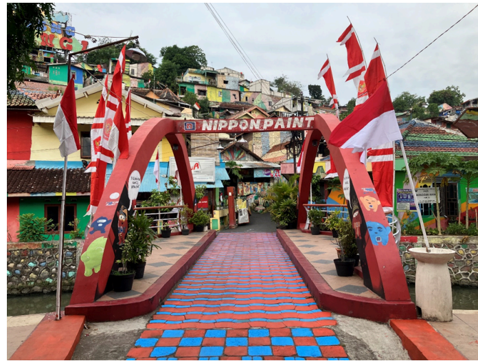
Figure 9. Before (upper) and after (lower) repainting the bridge on Jl. Wonosari 5. Source: Taken by Kawata on Aug. 6 and 7, 2024.
