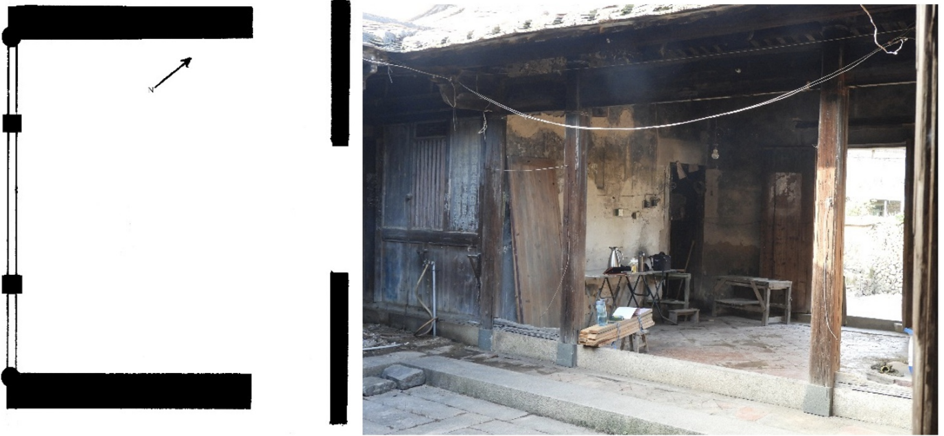
Figure 10. Room 5, the patio.
