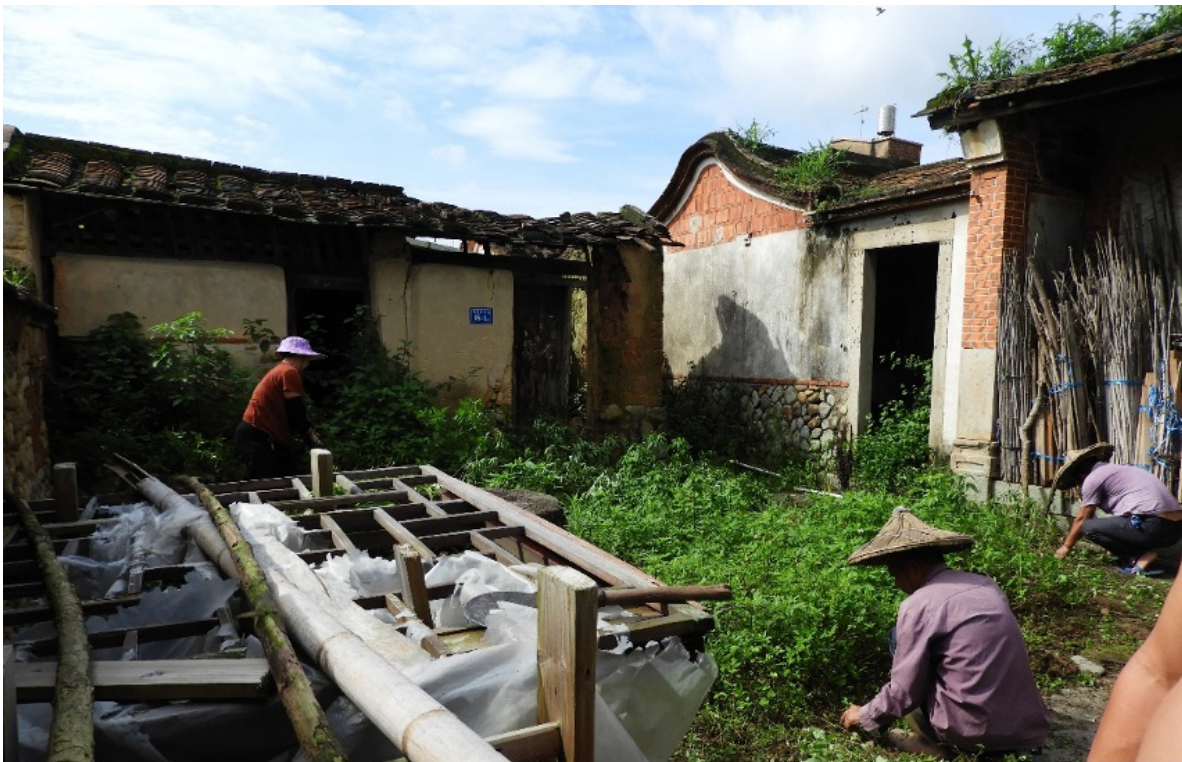
Figure 4. Clearing the vegetation in House unit 1 the front-yard
