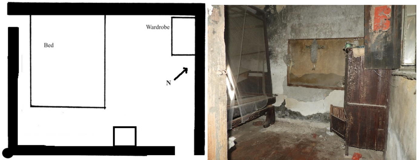
Figure 11. Room 6 with its abandoned furniture.
