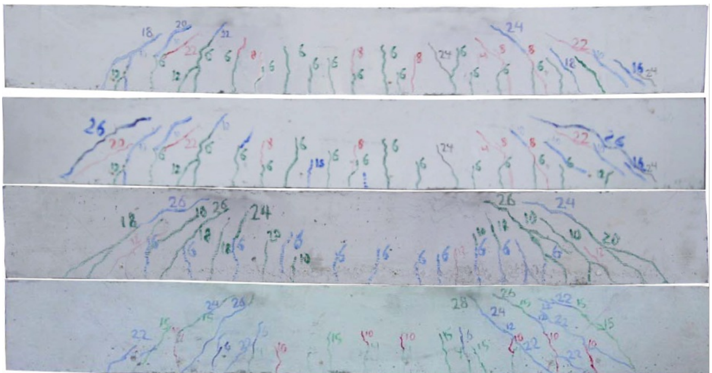
Figure 10. Appearance of cracks for the beams subjected to ultimate loads ( f_c=90 MPa)
