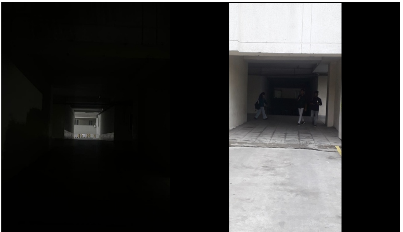
Figure 32. Road leading to parking with zero lux(left), same area(daytime)
