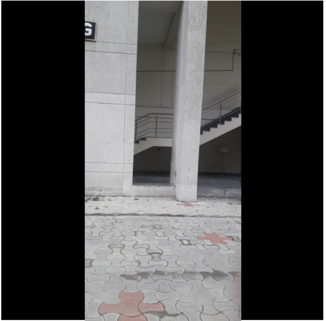
Figure 34. Open spandrel space below stairs leading to the central library
