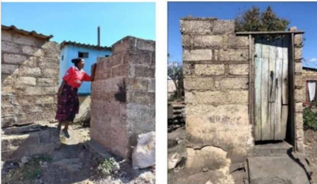
Image 2. 2A: Woman demonstrating how people peep inside her toilet, 2B: A toilet without roof and peepholes on doors. (Source- K Tembo)
